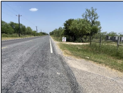
Photograph 14 – View looking east at the directional sign situated along FM 490 directing members of the public to the Hargill pop-up event.
